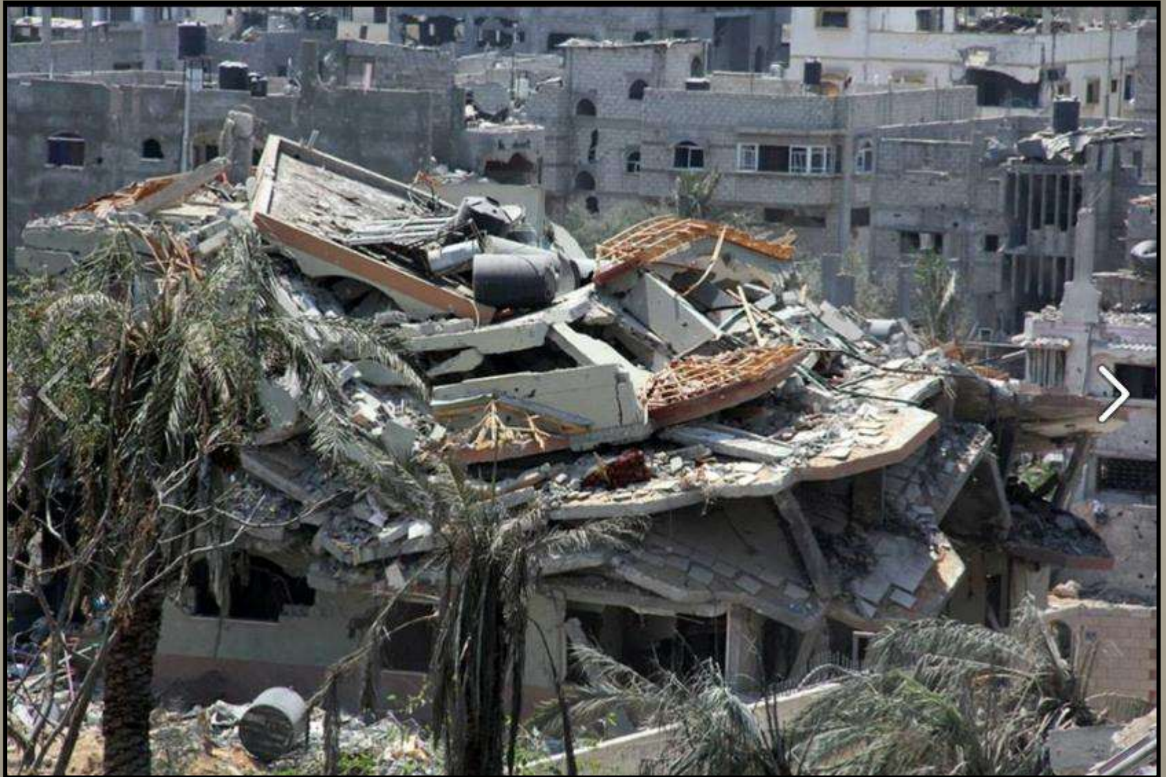
This building was probably hit by a implosion bomb
